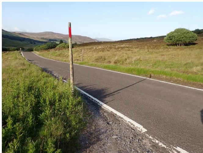
Looking NE-ENE from photo point
